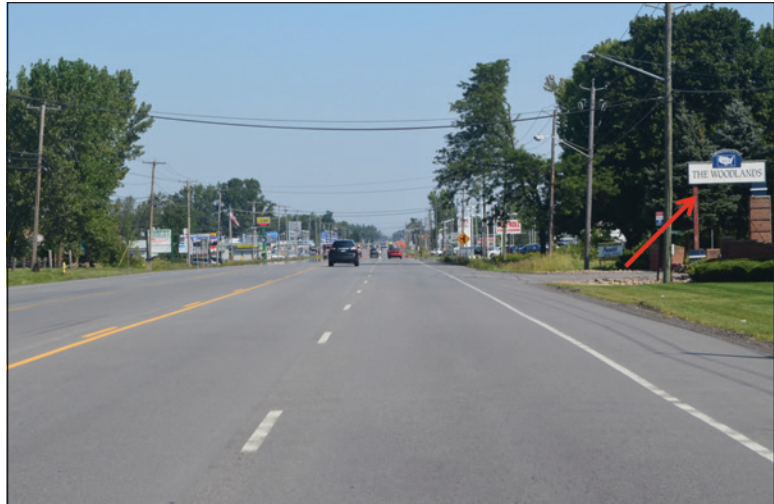
Figure 1 NY Route 78 looking northbound.
