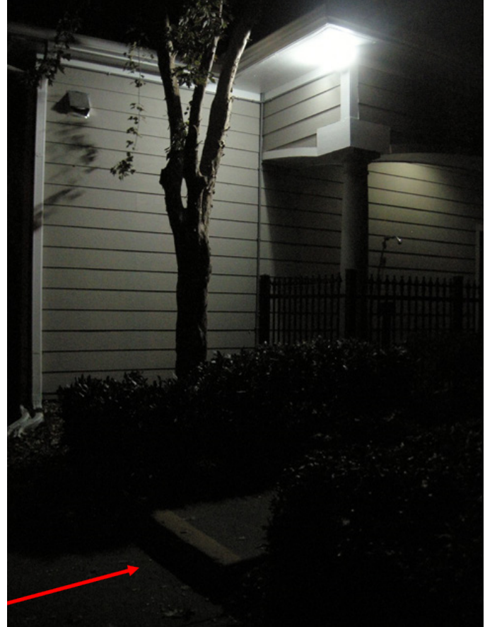
Figure 17 Primary illumination for walkway step down (arrow) at time of inspection
