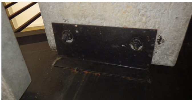
Figure 3 Concrete stair tread attachment to steel frame.
