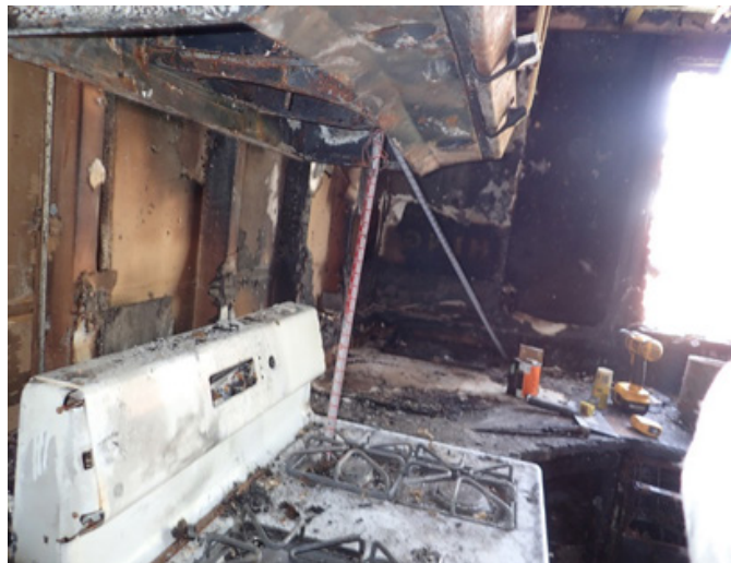
Figure 8 Reconstructing the range hood.
