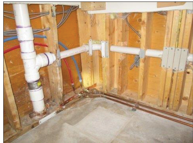
Figure 5 Kitchen walls removed, exposing piping.
