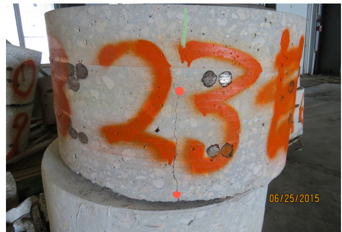
Figure 8 Concrete core with excessive flexural cracking.
