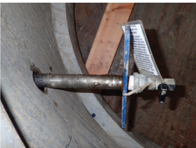
Figure 21 Test cavity bleed-off tube and valve.
