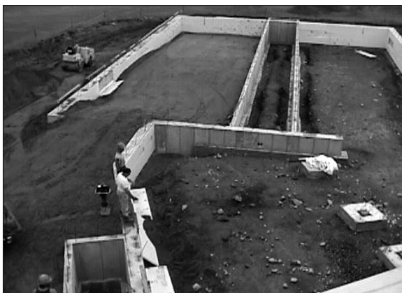
Figure 4 Elementary School Foundation with Initial Lift of Substitute Material
