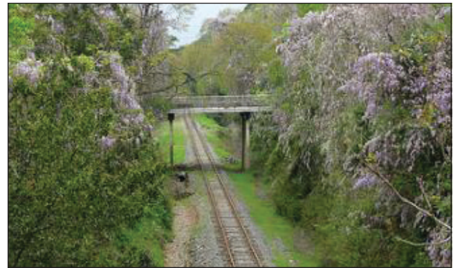
Figure 1 Vehicle bridge over Norfolk Southern Railroad.
