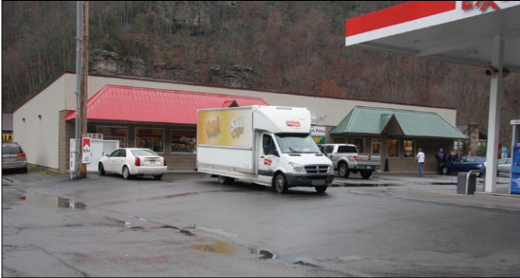
Photo 5 Completed Store Front
