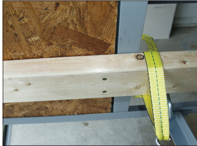
Figure 7 nailed installation of guardrail
