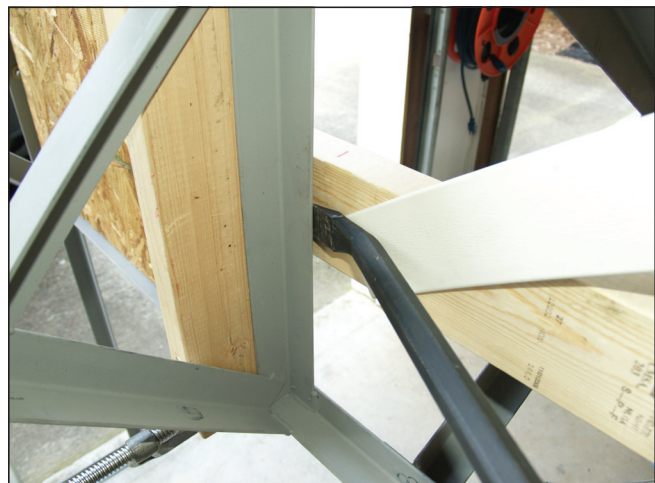
Figure 8 crowbar removal of guardrail
