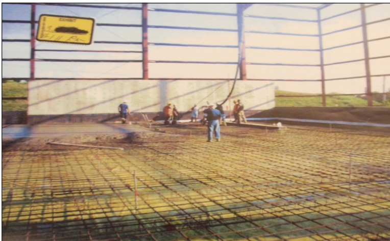
Figure 5 Overall View of the Jobsite.
