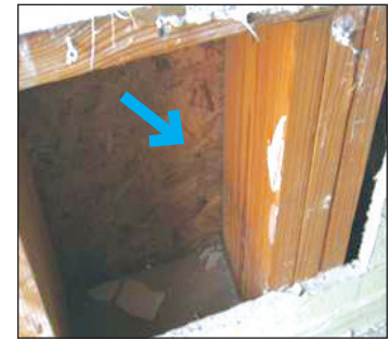
Photo 3 View From Within Wall Cavity
