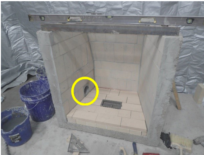
Figure 8e Dry-fit hearth refractory and log lighter kit. Combustion air kit ducting (circled).
