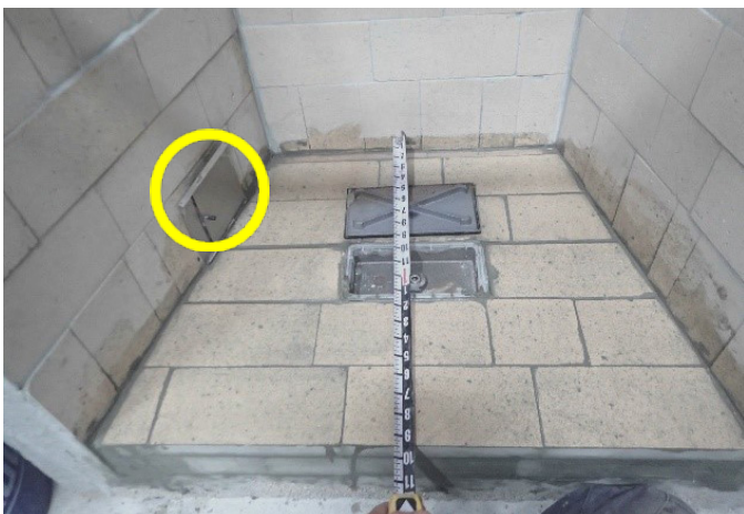
Figure 8f Constructed to match incident installation. Combustion air kit discharge register door (circled) near rear of the firebox and flush with the hearth.
