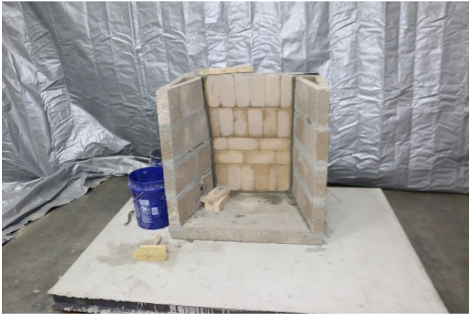
Figure 8d Firebox construction and wall lining refractory installation.
