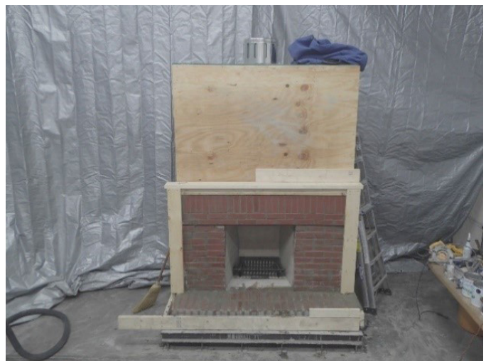
Figure 8i Chase walls, hearth extension, surround and mantel construction.
