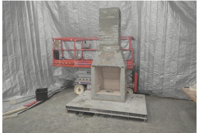
Figure 8g Smoke dome, damper, and masonry chimney construction in progress.
