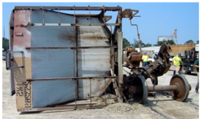
Figure 1 Rail car derailed from the tangent track (left); another view of the derailed rail car (right).
