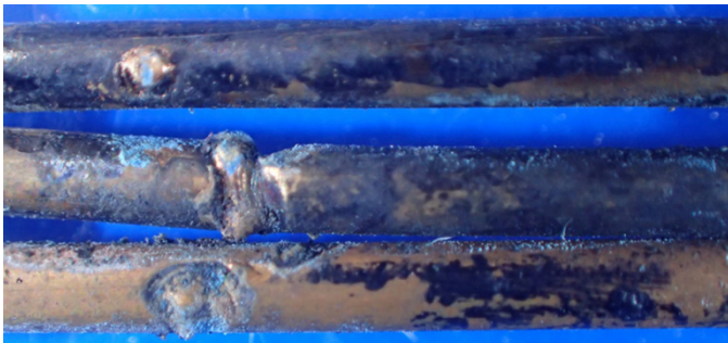
Figure 4 Example of electrical conductor arc melting damage 26 .
