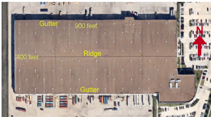
Figure 1 Aerial view of the subject warehouse.
