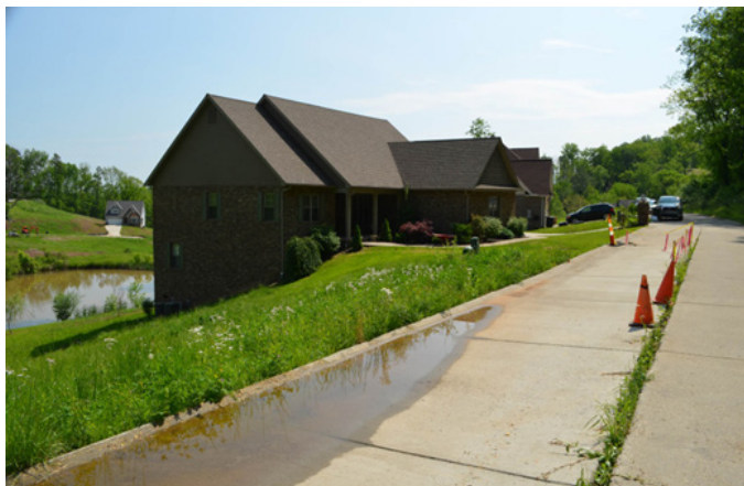
Figure 5 Elevation relief from street to rear of home was approximately 20 feet along left side.
