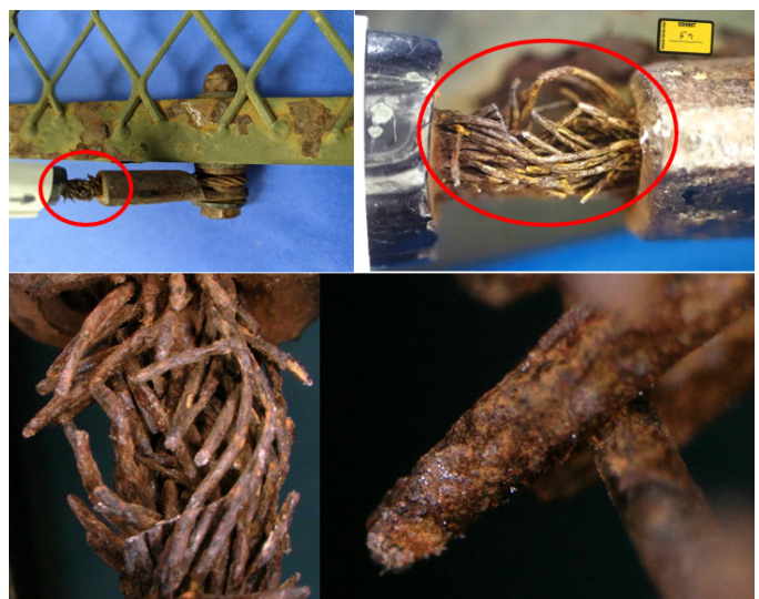
Figure 5 Right-side cable foot platform attachment and the frayed segment between the eyelet and crimp with focus on elongated strands, characteristic of ductile failure.
