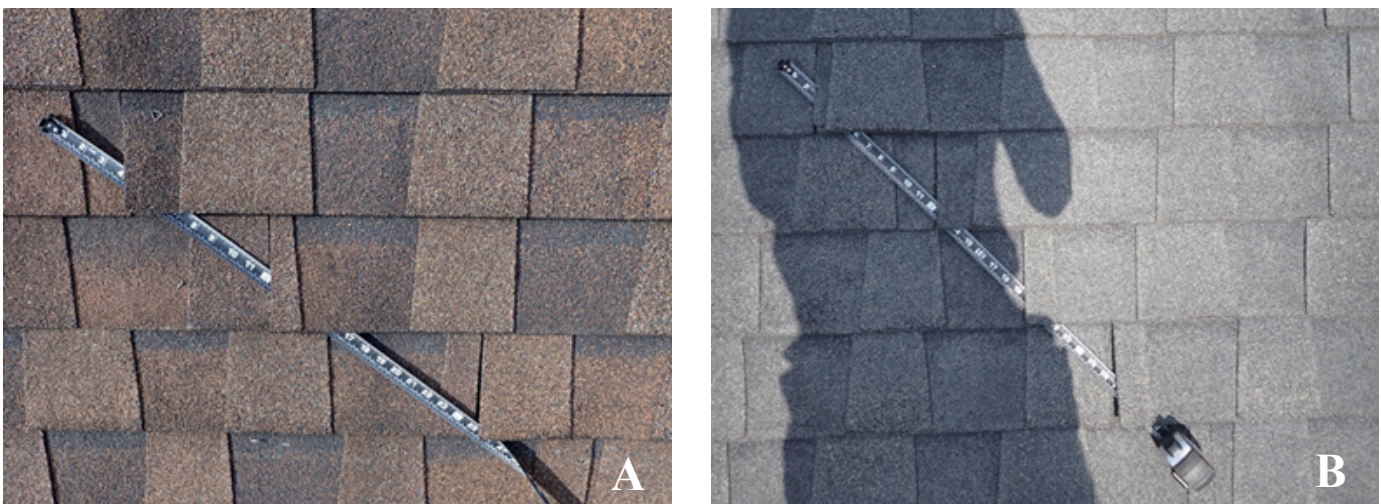
Figure 4 Shingle diagonal debonding pattern.
