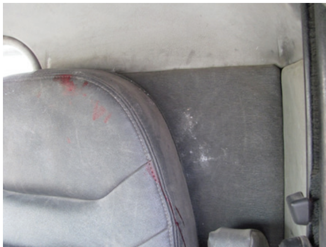
Figure 20 Concrete fragments along panel behind driver’s seat.
