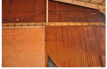
**Figure 8** Metal gate (internal surface) — intense corrosion.
