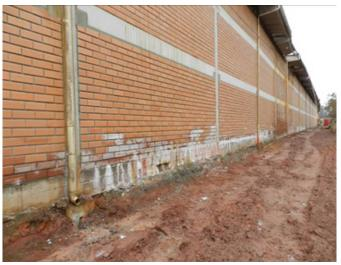
Figure 7 By-products of the reaction on the outer face of the warehouse wall.
