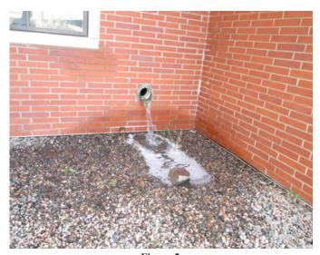
**Figure 5** Substantial completion observation (July 24, 2018) showing storm drainage water accumulation at the backfill zone of the foundation.
