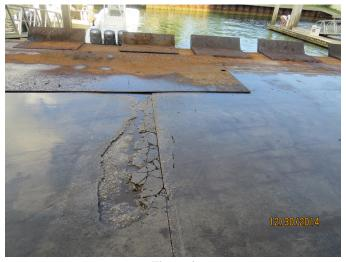
**Figure 6** Runway surface spalls and cracks.
