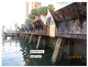
Figure 3 Marina bulkhead king pile and slab system.
