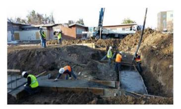
Figure 3 Owner-provided photograph (Nov. 6, 2015), showing concrete placement for footings. Note that the dowels necessary to connect the footing to the foundation walls are not in place prior to the pour. The stabbing of dowels is a violation of the code, and was strictly forbidden by the structural engineer of record.
