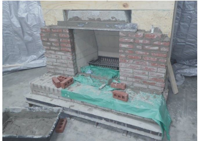
Figure 8h Chase walls, hearth extension, and surround construction.
