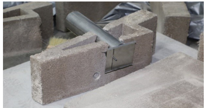
Figure 8b Combustion air kit installation and through hole for gas line to log lighter.
