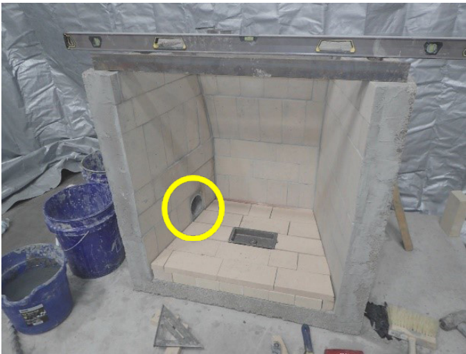
Figure 8e Dry-fit hearth refractory and log lighter kit. Combustion air kit ducting (circled).
