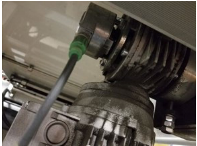
Figure 12 One of the position sensors that regularly failed shows intact cabling and shielding.
