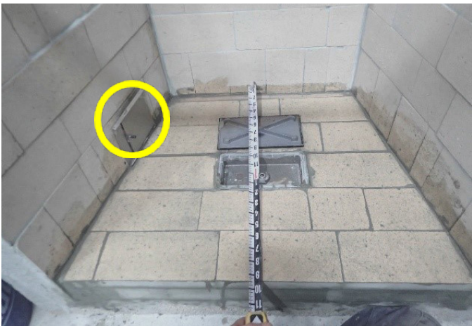
Figure 8f Constructed to match incident installation. Combustion air kit discharge register door (circled) near rear of the firebox and flush with the hearth.
