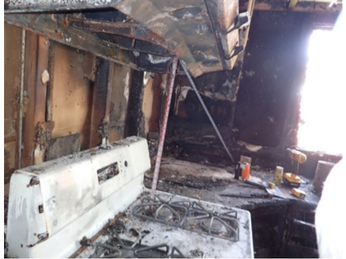
Figure 8 Reconstructing the range hood.
