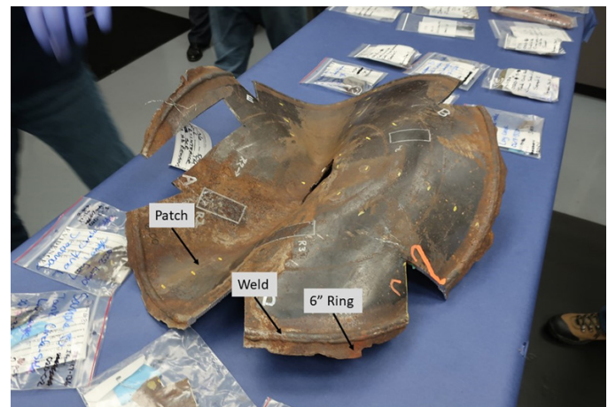
Figure 9 Repaired bottom cap with the 24-inch patch after the failure (photograph taken by Kineticcorp).
