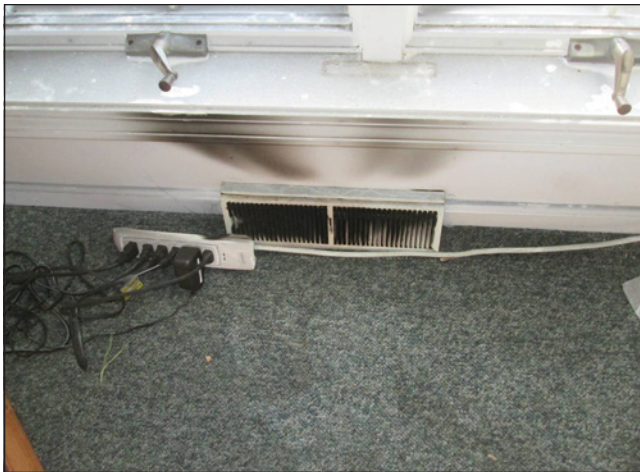
Figure 7 Soot damage.
