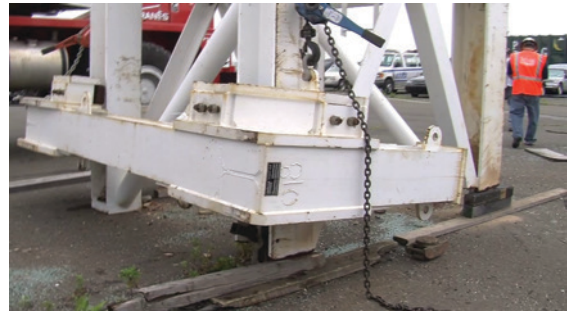
Collar tie section completely supported on crane tower.
