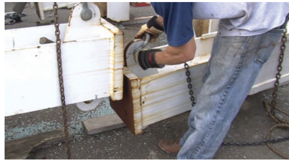
Second collar tie being setup for bolt up alignment.
