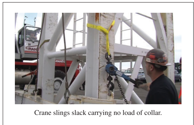
Figure 38 Collar tie half transferred from the crane to slings.
