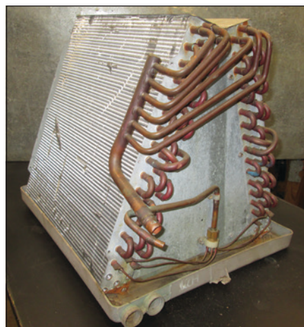
Figure 4 Evaporator coil.
