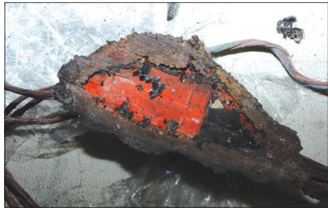
Figure 15 Plug (black) and socket (orange) showing minimal damage.
