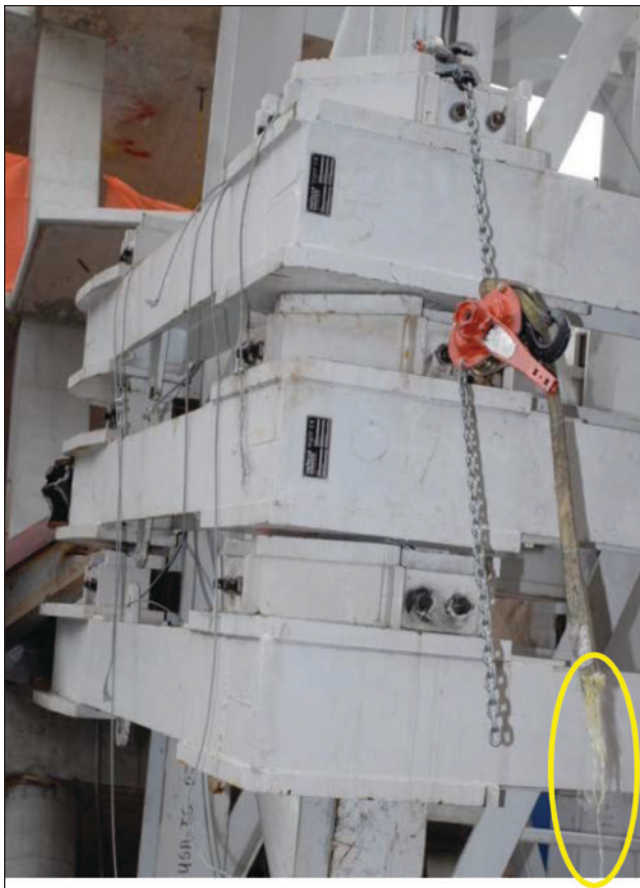
Figure 30 SW corner with Ex_Lift sling 1A. Visibly extended fibers are evidence of slow-speed failure.
