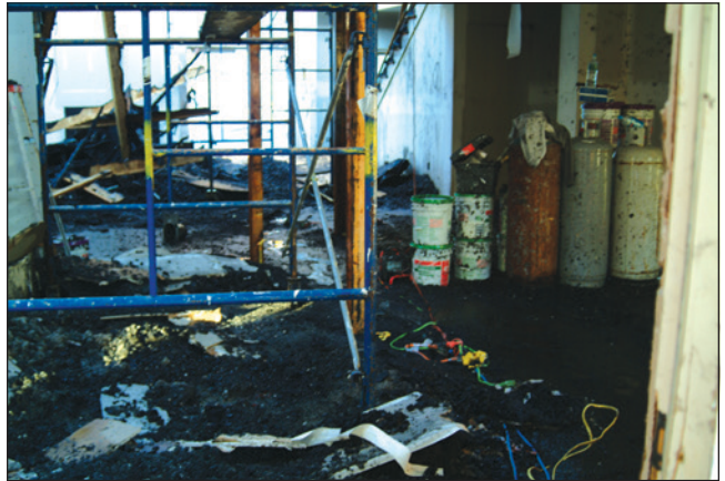
Figure 6 Paint cans and propane tanks.
