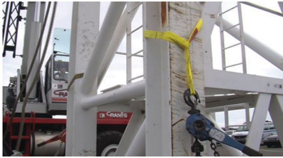
Slings from support crane removed from collar tie.
