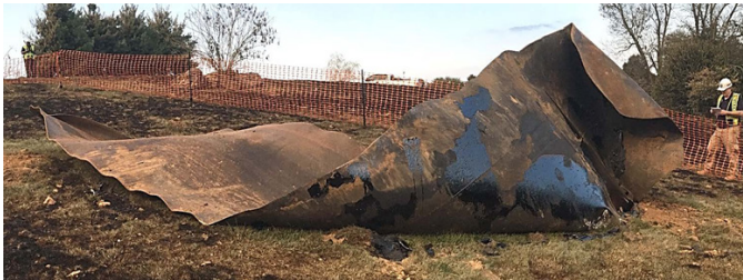
Figure 5 The 33-foot-long segment of pipe that was ejected as a result of the explosion 4 .
