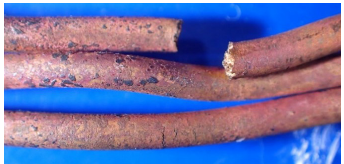
Figure 7 Example of electrical conductor mechanical damage 26 .
