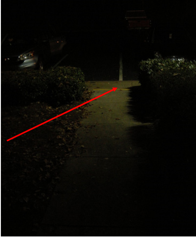
Figure 16 Walkway at night looking toward single step down (indicated by arrow).
