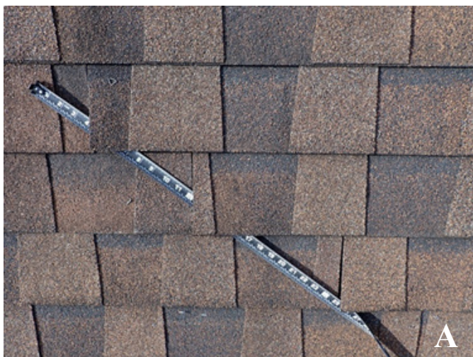
Figure 4 Shingle diagonal debonding pattern.
