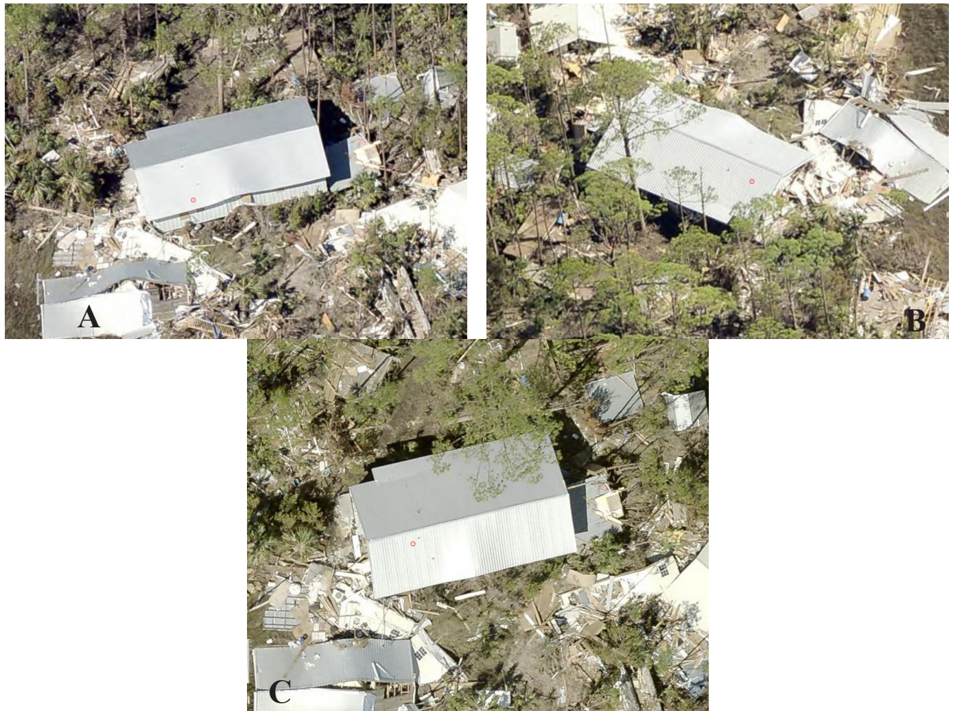
Figure 20 Displaced structure — approximately 1,780 feet northeast from its original location: (A) right elevation view, (B) left elevation view, and (C) top view (all figures courtesy of Eagleview [54]).
