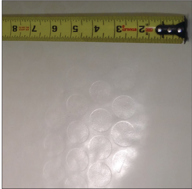
Figure 4 Slip-resistant features along bottom of subject bathtub.
