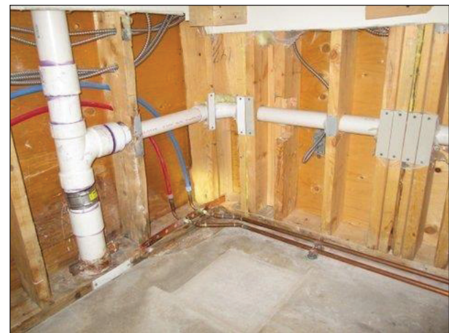
Figure 5 Kitchen walls removed, exposing piping.
