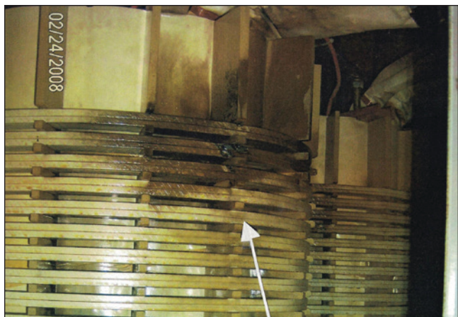
Figure 2 Transformer short circuit #1.
