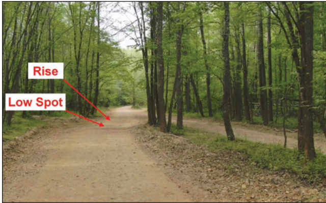
Figure 12 Case B: Accident site.
