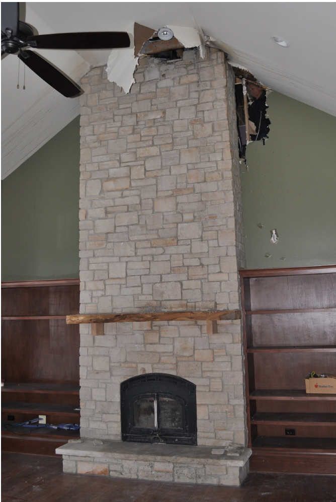
Figure 9 Family room showing fireplace and chase.
