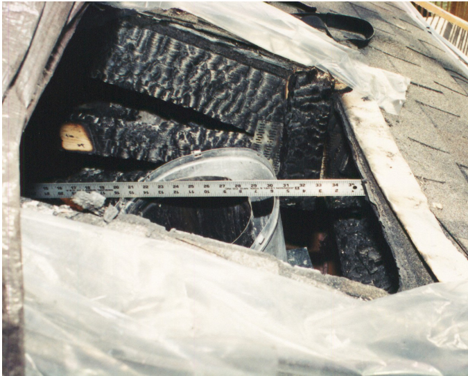
Figure 4 Top of chimney assembly in house attic.
