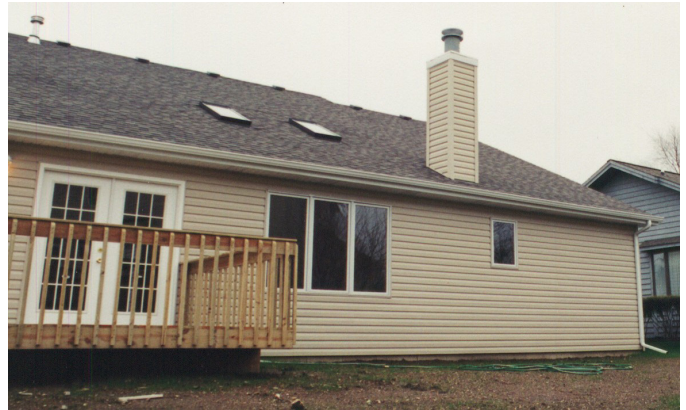
Figure 6 Exemplar house showing chimney chase.
