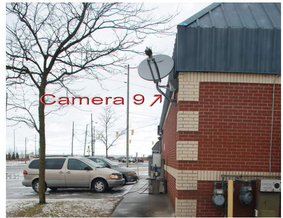
Figure 14 Camera 9 was mounted at the southwest corner of the restaurant.
