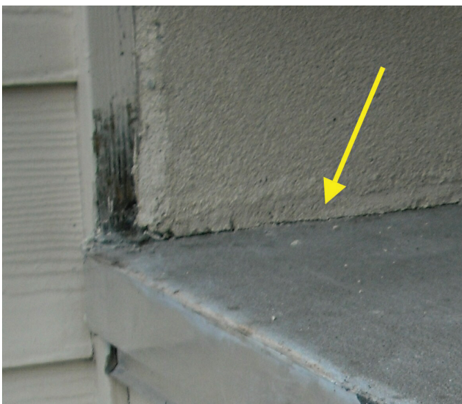
Figure 9 Stucco contacts patio.
