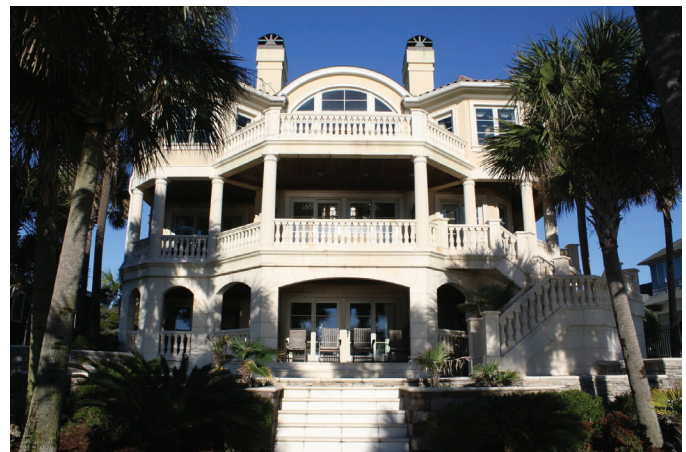
Figure 1 Oceanfront elevation of subject residence.
