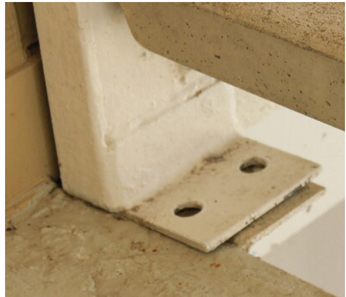
Figure 7 Missing bolts.
