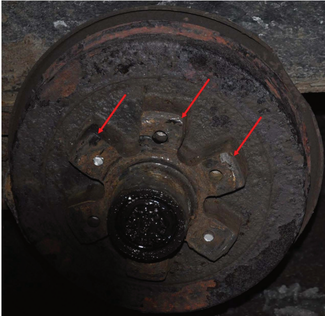
Figure 5 Accident trailer left front hub at time of accident.
