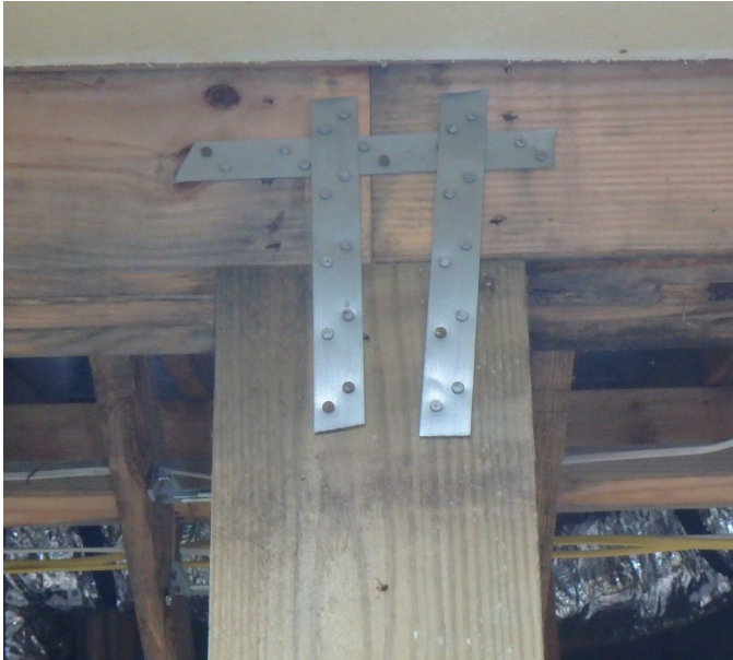
Figure 2 Defective connection.
