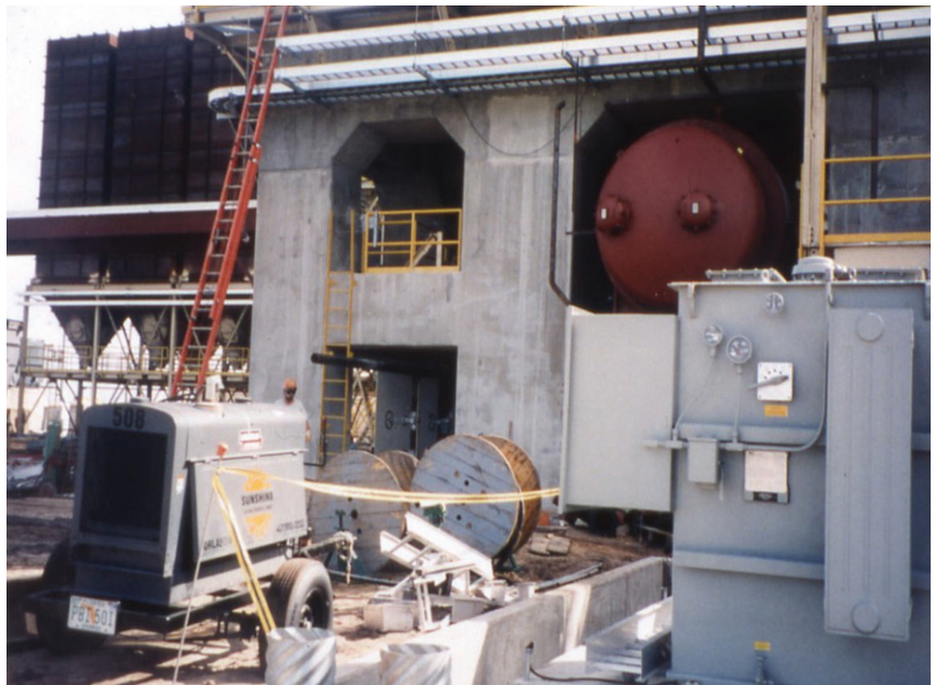
Figure 10 View of repaired STG structure.
