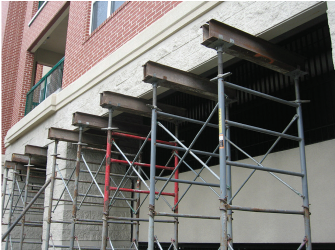
Figure 13 Over-spanded headers.
