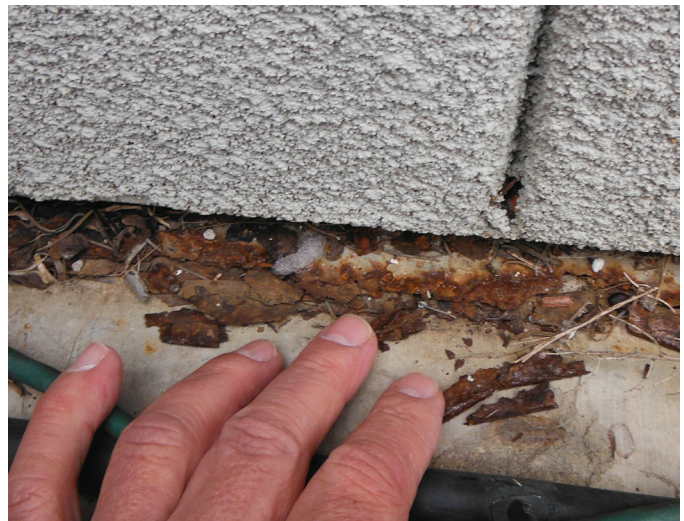
Figure 16 Rusted flashing.
