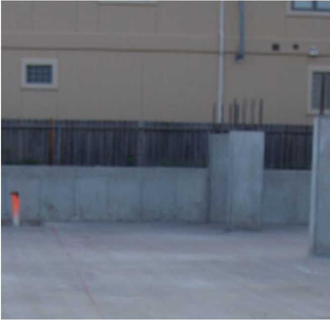
Figure 19 Different site condition.
