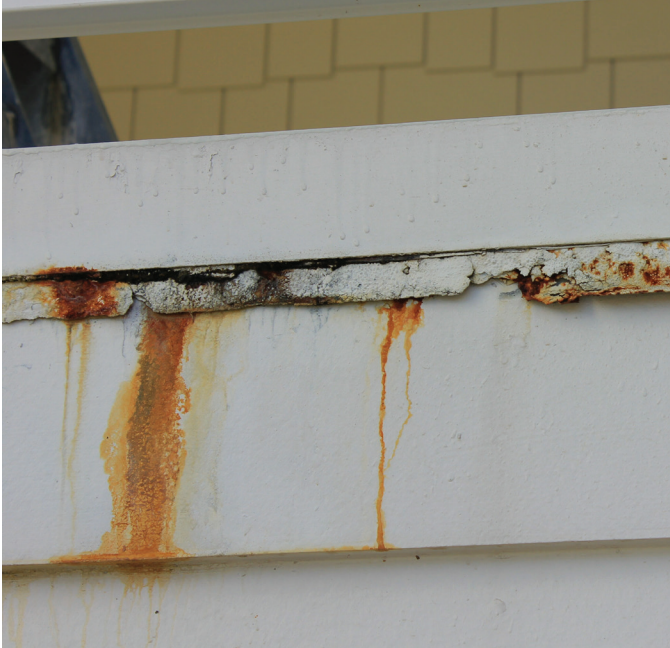
Figure 17 Rusted flashing.
