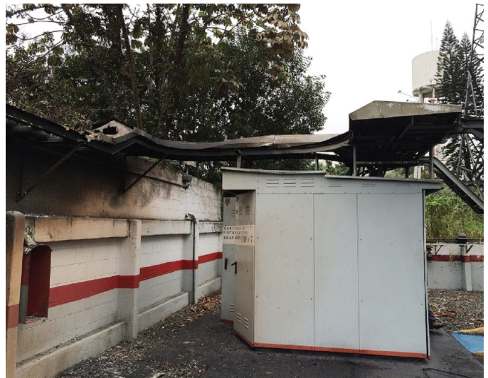
Figure 9 Cable tray with cable splice failure.
