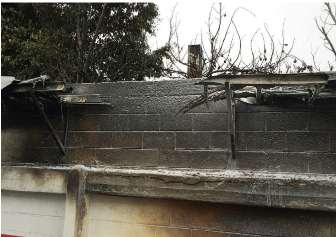
Figure 7 Cable tray with cable splice failure.
