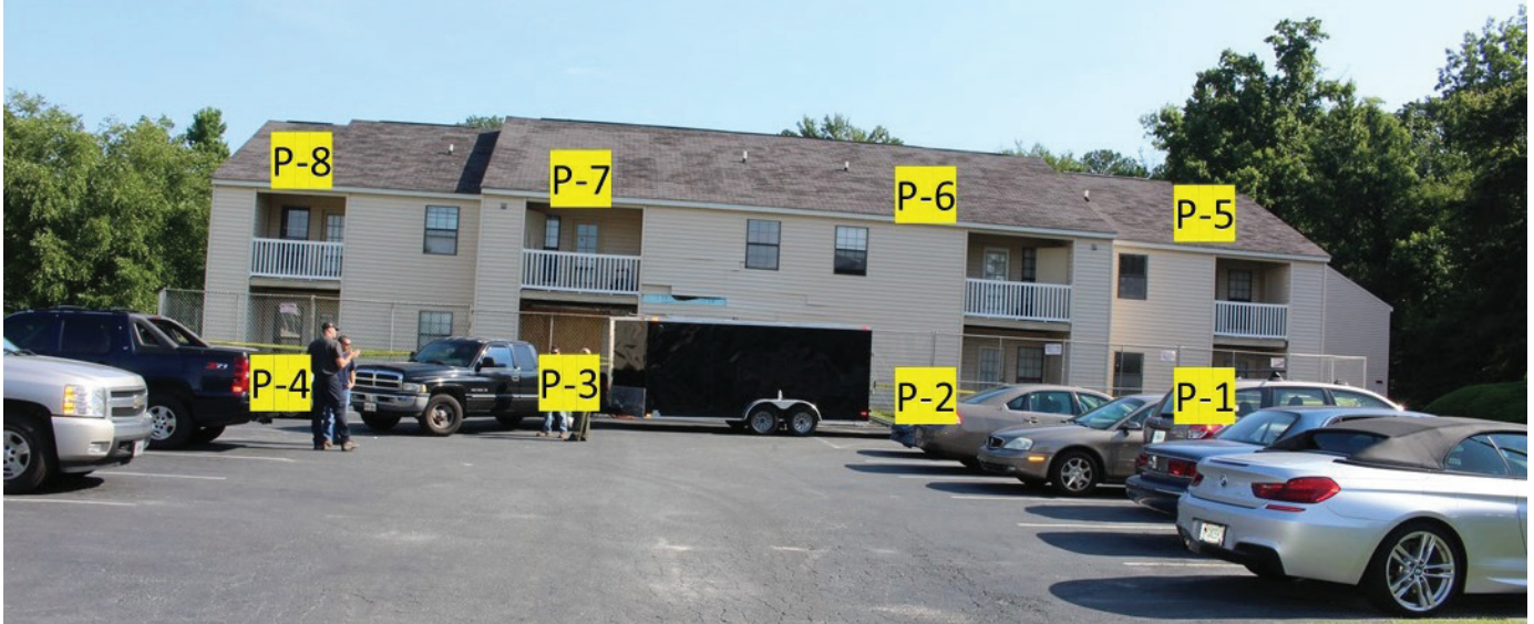
Figure 2 View from the rear (south side) of Building P.
