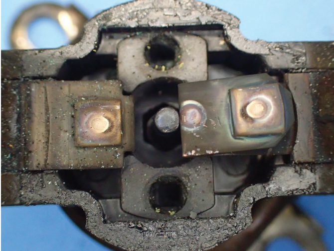
Figure 14 Contacts of gas dryer safety thermostat.
