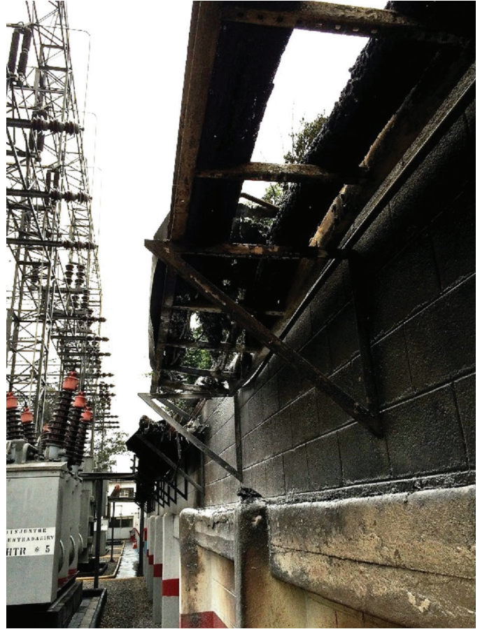
Figure 8 Cable splice failure.
