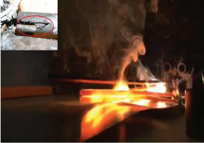
Figure 13 Heater arcing due to overheating damage. https://youtu.be/KJ8sIBma22o
